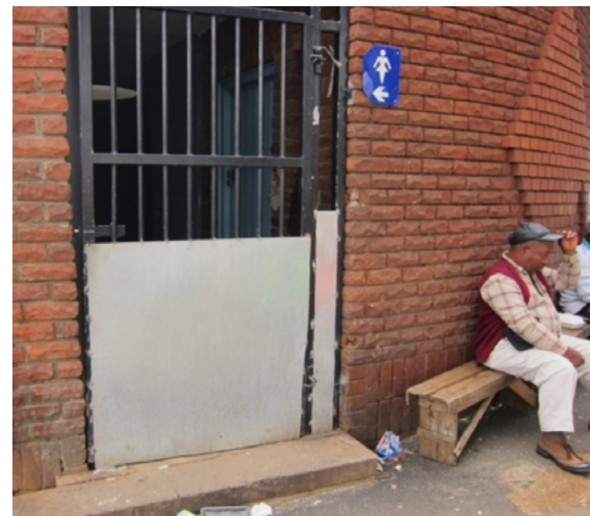
Neglected washroom facilities in Warwick Junction. Photo: AeT
