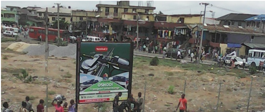
The demolished Owonifari Market, Oshodi, to make way for the 'Oshodi Transport Interchange' (FIWON, August 2016).
