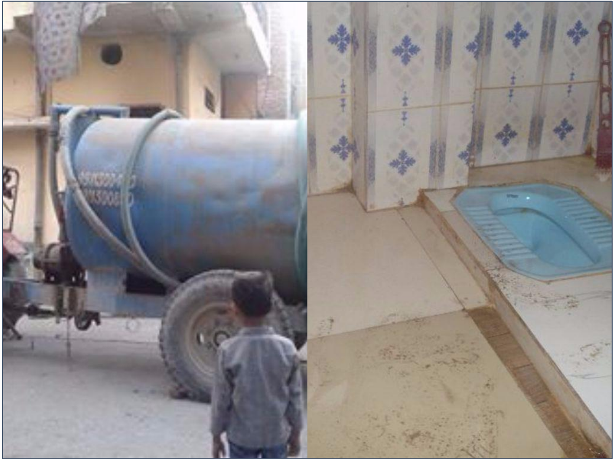
Figure 29 Pit toilet has been installed at my house and the septic tankers come for pumping (cleaning the pit) it out when it gets choked-Anjali
