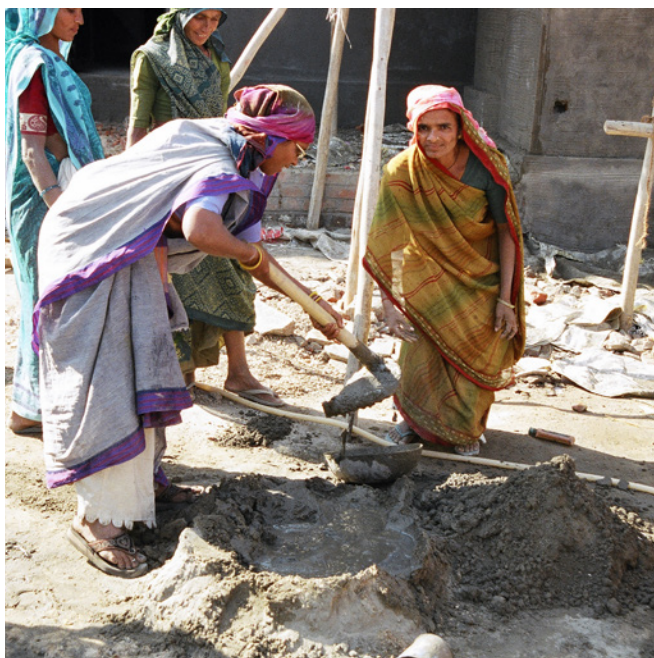
Construction workers in Ahmedabad. Photo by WIEGO
