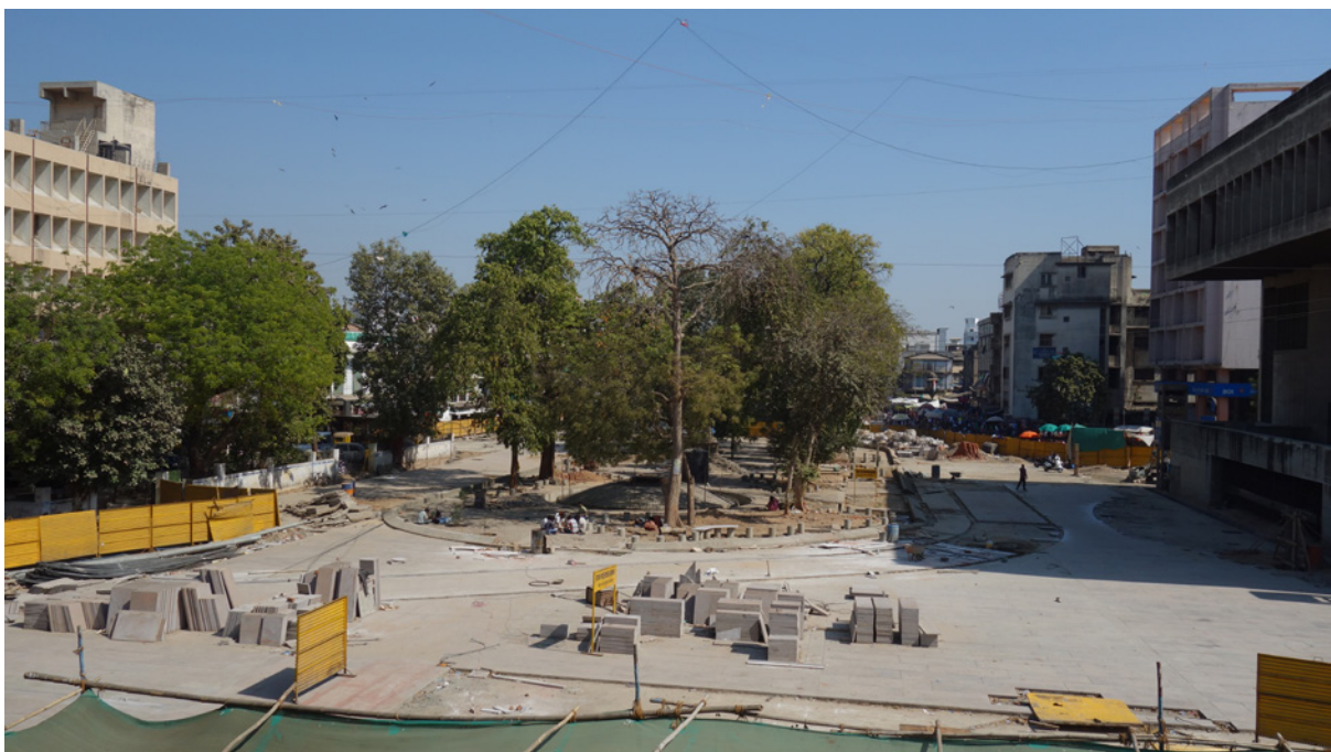
Cordoned-off area for plaza development, 2013.
